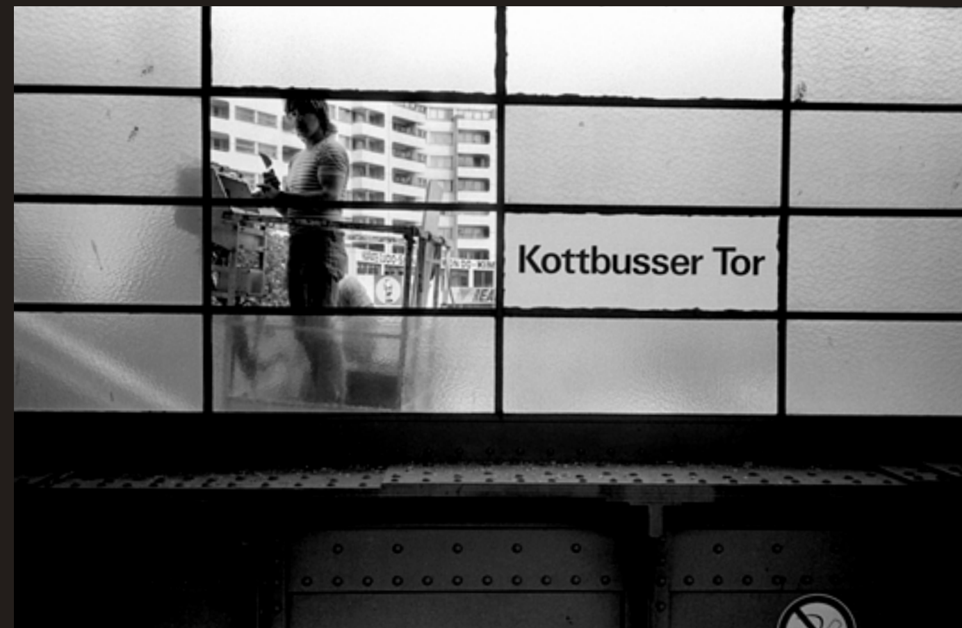
A worker repairs windows at the Kottbusserdam station, located near the center of Kreuzberg.
