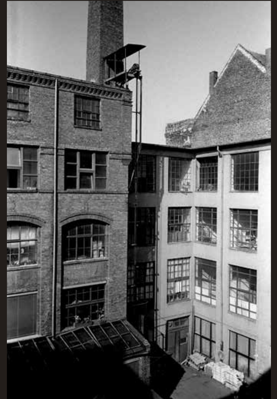
Many of Kreuzberg's residential buildings have small manufacturing companies occupying the bottom floors.
